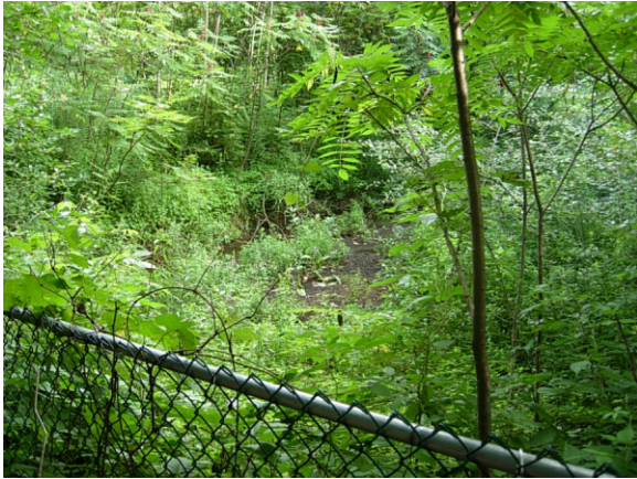
The existing Winding Brook detention pond was filled in with sediment and overgrown with vegetation.
