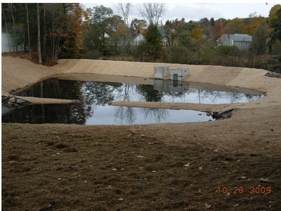
Photo of the Winding Brook shortly after reconstruction. The size of the pond was increased to provide detention of large volumes of stormwater runoff.
