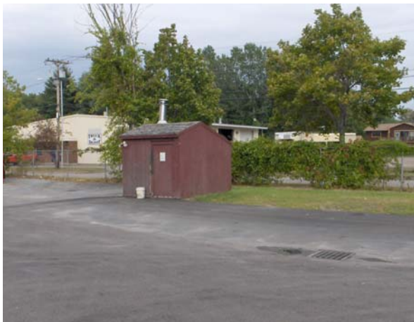
Reconstructed vehicle washing area
