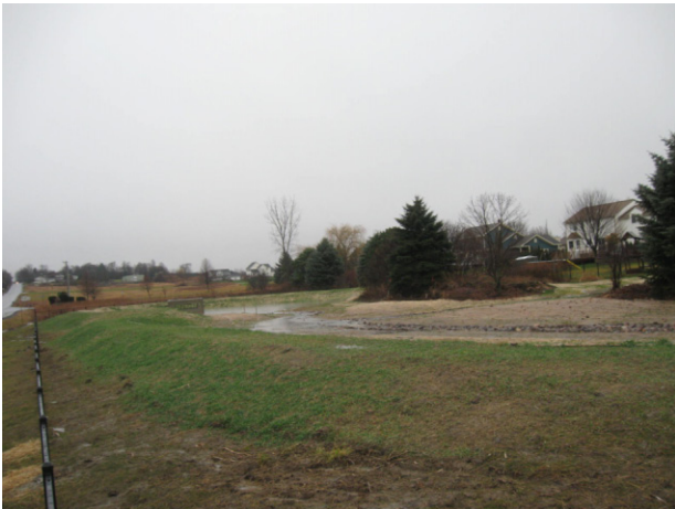
View of pond berm shortly after construction.
