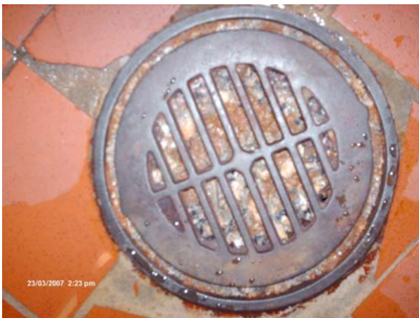
Meat department floor drain.
