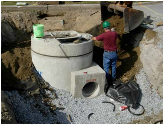
City staff backfilling around new swirl separator on Gregory Drive
