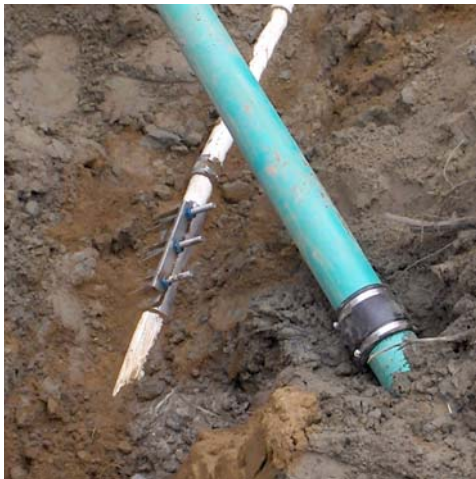
Repaired 2" sewer line underneath stormwater piping
