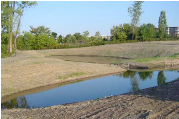
New detention basin installed as part of the Farrell Street project. Photo taken during construction.
