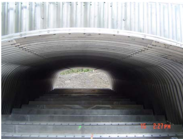
New detention basin installed as part of the Farrell Street project. Photo taken during construction.
