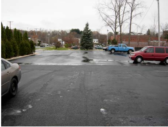
Porous Asphalt installed as part of the Farrell Street project (foreground).
