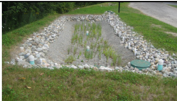
Photo of the gravel wetland after initial planting.
