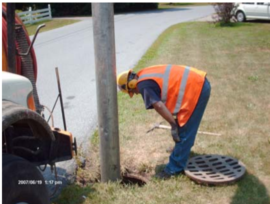
Cleaning a storm drain with the vacuum truck
