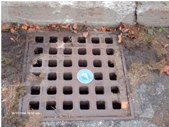
A storm drain in South Burlington
