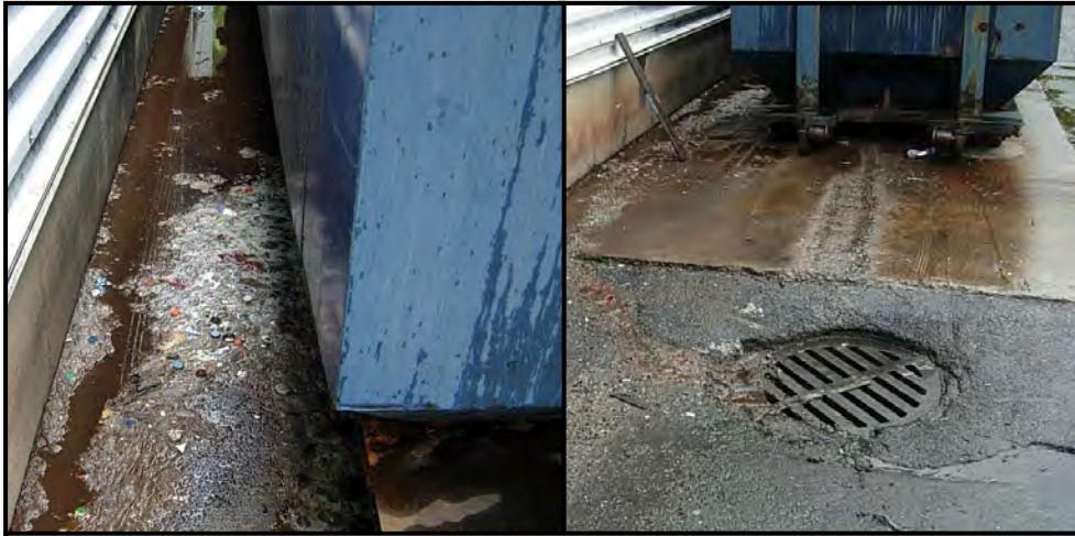
Out of date soft drinks were being disposed of in a compacting dumpster at a warehouse facility. Spoiled fluids would leak out of the dumpster into a nearby storm drain.
