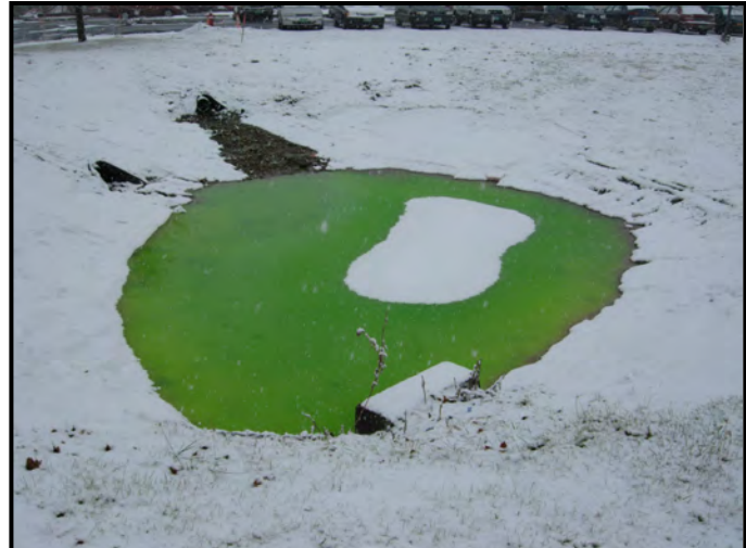
Propylene Glycol dumped down a storm drain collected in a stormwater detention pond located down stream.
