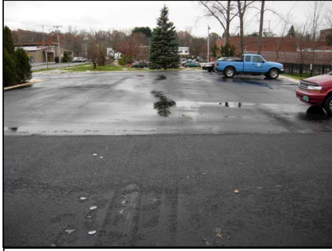
Pervious Asphalt installed as part of the Farrell Street Stormwater Project is visible in the foreground
